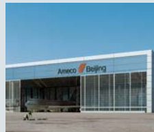
Ameco A380 Hangar Peking, China
